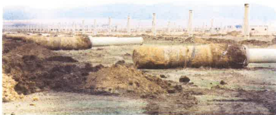
Abandoned Carrizo Plain's solar power plant (via Center for Land Use Interpretation )
